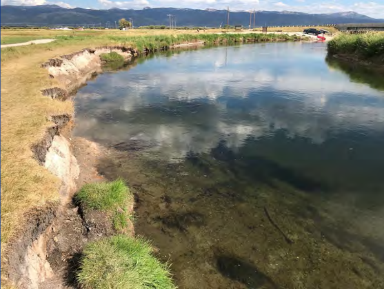
Eroding Bank at Boat Ramp Before
