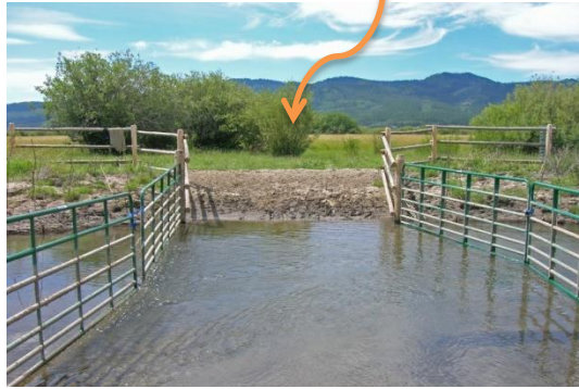
This hardened stream crossing for cattle on Trail Creek limits erosion and provides a single place for cattle to get across the stream.
