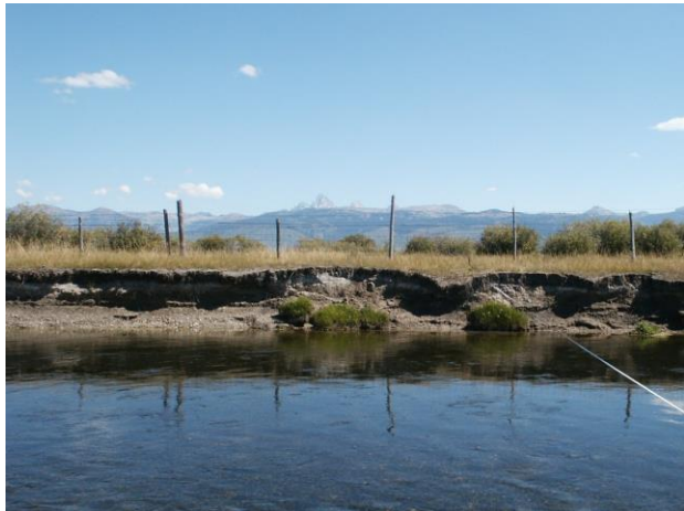
Before Conditions: Unstable and eroding stream banks, lacking vegetation.
