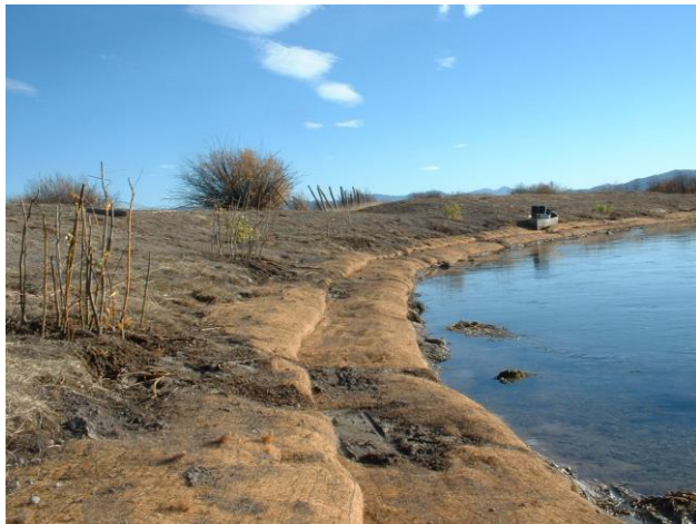
Bank reinforcement using coconut husk mesh/netting.
