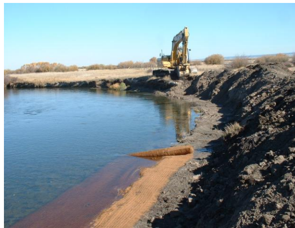
Constructing First Soil Terrace
