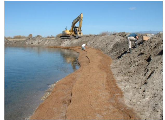
Constructing Second Soil Terrace: Stabilizes banks and reduces down cutting.
