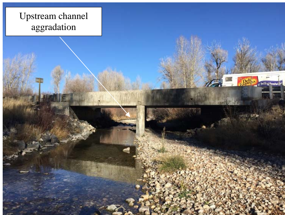
Figure 26. Photograph 24, deposition in river left bay of Highway 33 Bridge, Station 115+00 ft.
