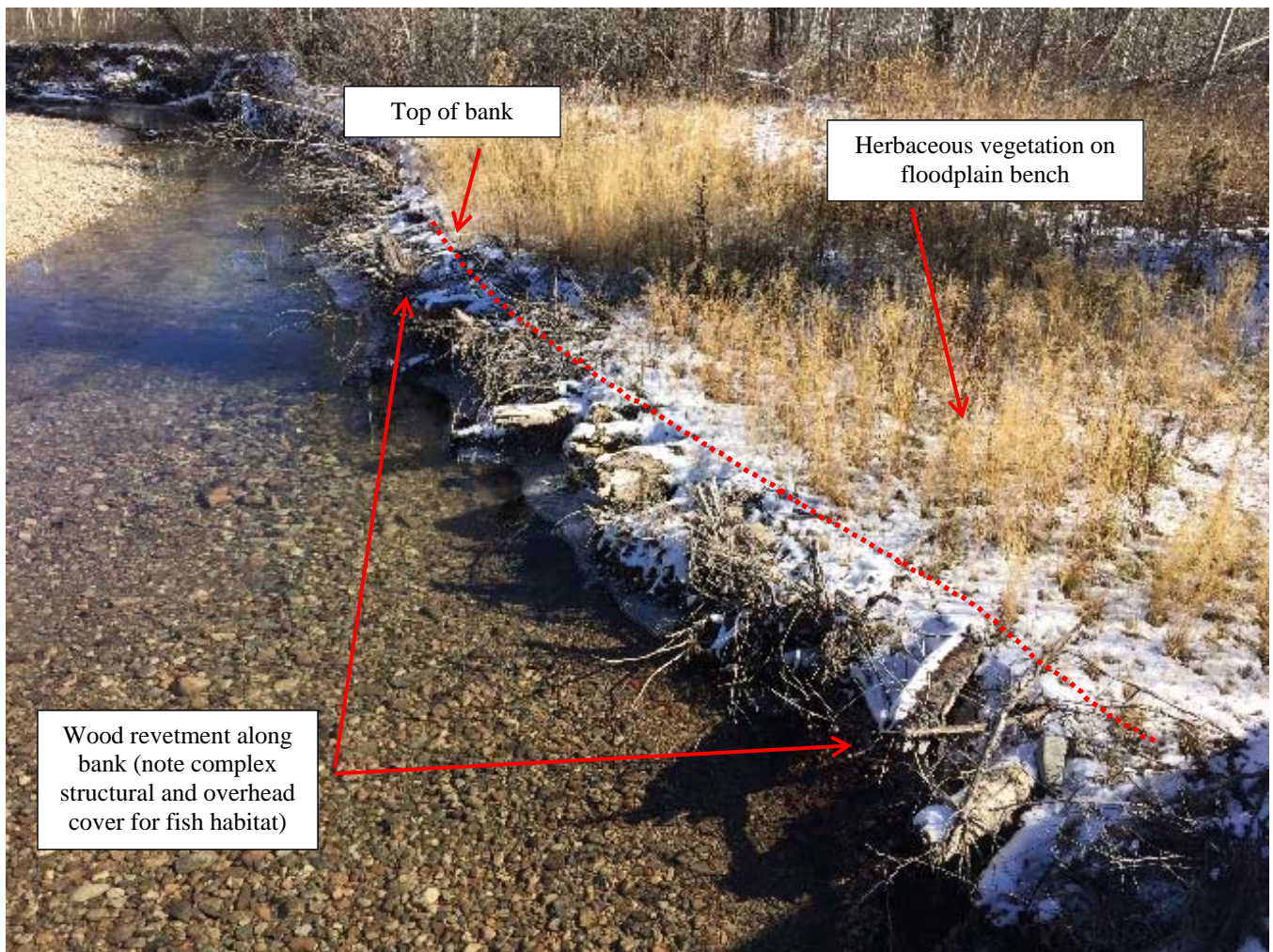
Figure 45. Wood revetment installed along river bank to prevent bank erosion, establish suitable channel width, and enable floodplain inundation.
