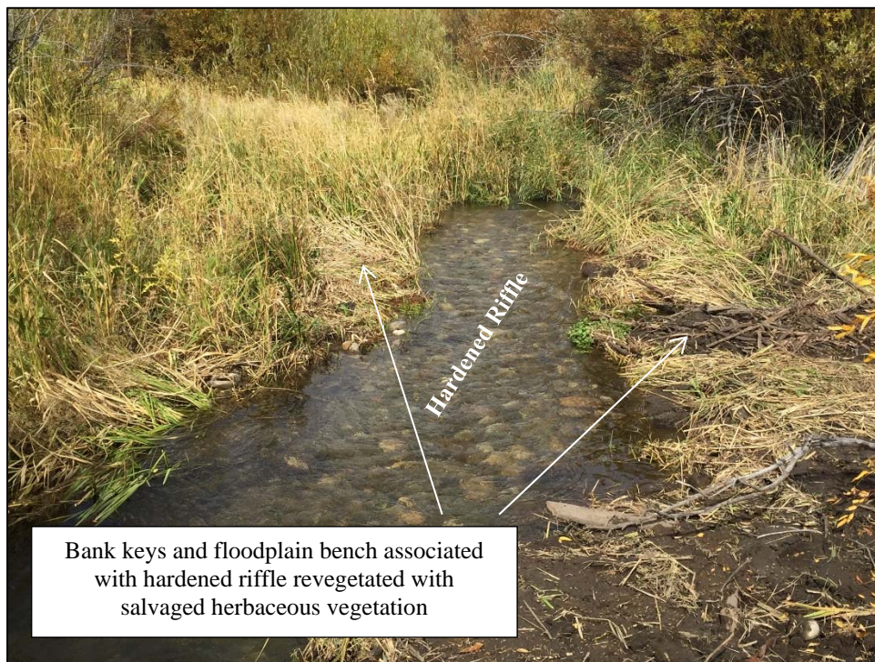
Figure 58. Photograph of installed hardened riffle grade control treatment.
