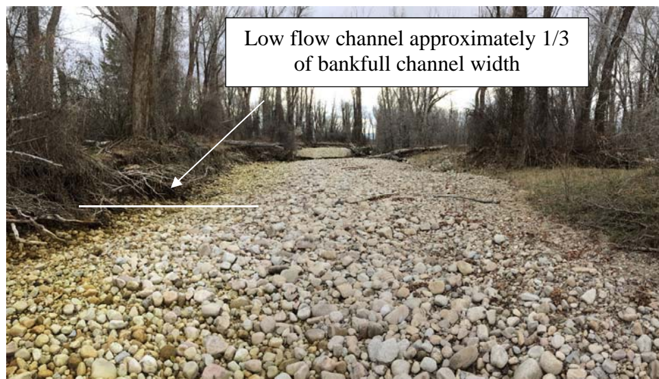
Figure 4. Photograph 2, relatively functional channel geometry with vegetated banks and low flow channel downstream of Cemetery Road Bridge at Station 2+00 ft.
