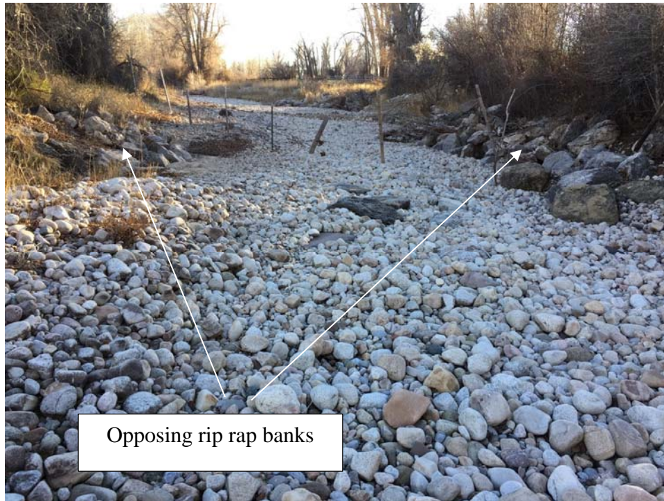
Figure 15. Photograph 13, bank armoring through rip rap installation on opposing stream banks, Station 64+00 ft.
