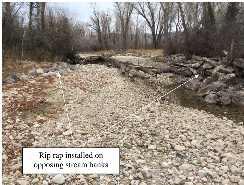
Figure 14. Photograph 12, bank armoring through rip rap installation on opposing stream banks, Station 59+00 ft.
