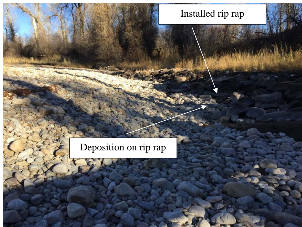
Figure 22. Photograph 20, sedimentation, pool filling, and channel aggradation covering installed rock rip rap, Station 93+00 ft.
