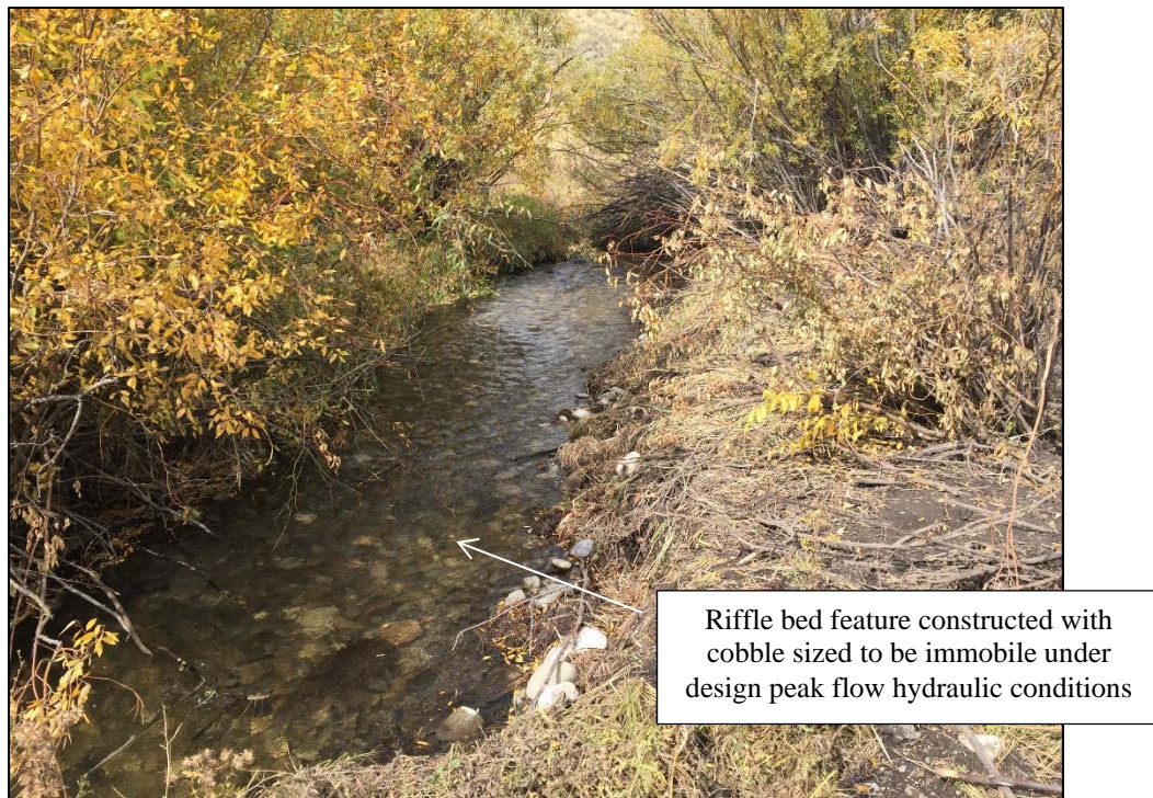
Figure 57. Photograph of installed hardened riffle grade control treatment.
