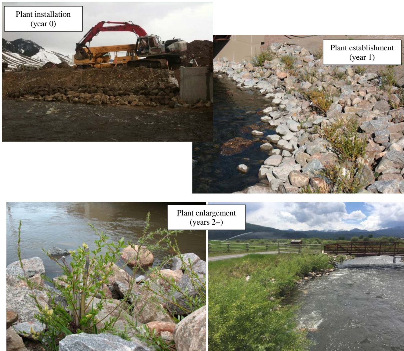
Figure 48. The rock revetment with bioengineering treatment incorporates vegetative material installed throughout the placed rock (top left). Installed vegetation establishes in the first year after construction (top right) and continues to expand in the second year after construction (bottom). The vegetation eventually establishes a complex root system to reinforce bank stability, and develops a robust canopy to provide over-head cover and fish habitat in addition to shade and riparian structure.
