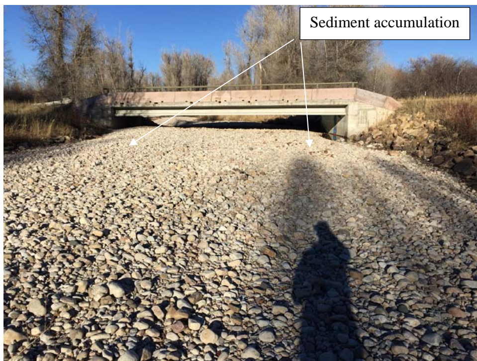
Figure 20. Photograph 18, high width/depth ratio channel and sedimentation/aggradation at Creekside Meadows Bridge, Station 87+00 ft.
