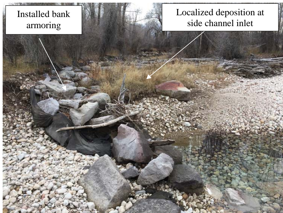
Figure 12. Photograph 10, bank armoring on the channel margin, with localized deposition that has filled the inlet to a side channel, Station 52+00 ft.
