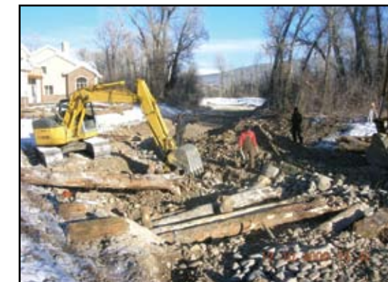
Restoration crews used buried logs to stabilize the stream banks and dissipate stream energy naturally.
