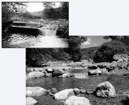
New fish-friendly irrigation structures open up migration corridors and keep trout in-stream, while delivering the water irrigators need.
