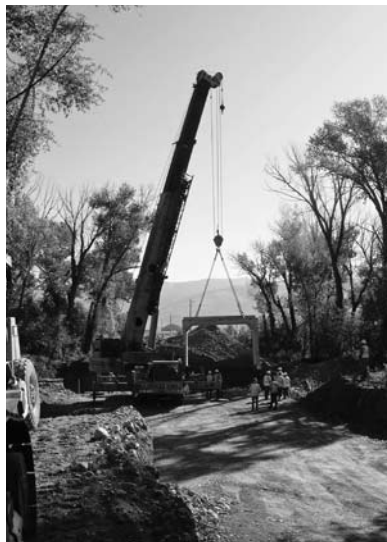
A large crane is used to "fly-in" a bridge section.
