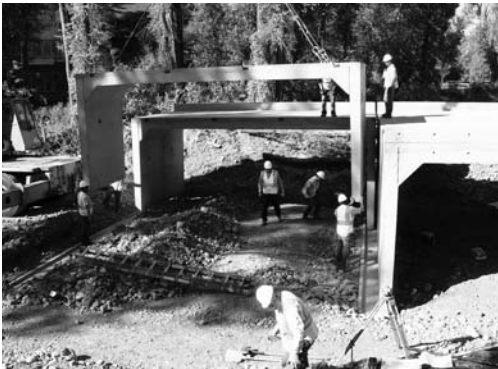
Teton County Road and Bridge crew places the middle section of the bridge.
