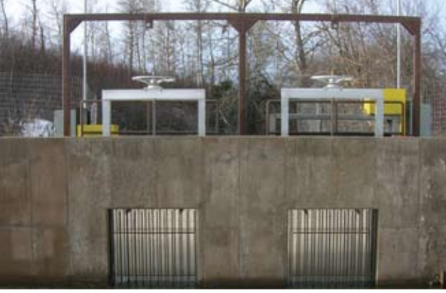
In a similar project, FTR built a fish-friendly diversion structure on Badger Creek.
