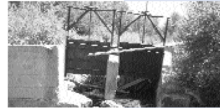
Current condition of the irrigation splitter on Badger Creek.
