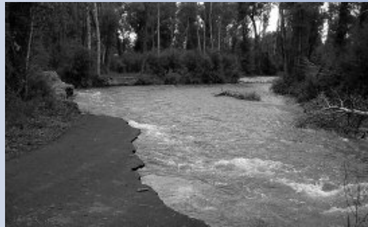
Looking upstream from the eroding Creekside bike path during the spring of 2006.
