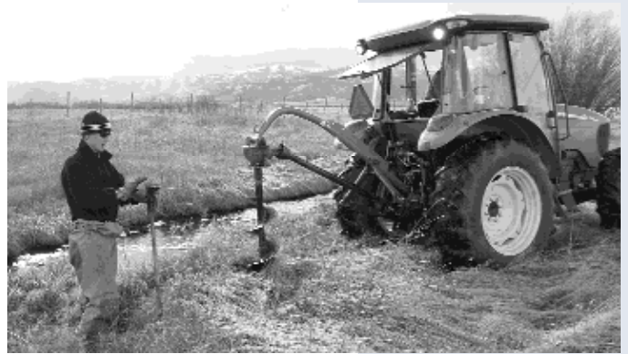
Ryan Colyer clears the way for the auger
