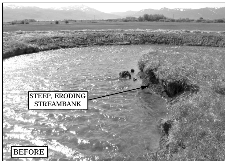
A steep, eroding streambank is replaced by a terrace covered with wetland sod that constricts the channel and increases the velocity of the current.
