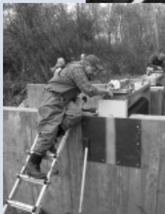
Top to Bottom: Installing one of two rotating screens (made by Intralox) into the new diversion structure on Badger Creek; After months of planning...the moment arrives, the screens are placed, and they fit!; Jeff Peterson (Bureau of Reclamation) installs a solar-powered motor that will drive the screens.
