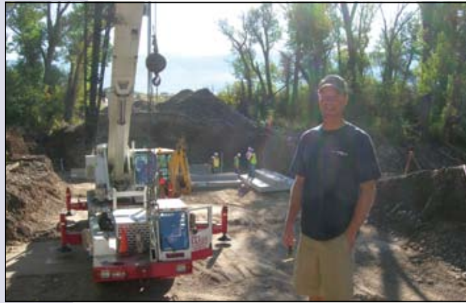
Mike Lien installing the new bridge on Teton Creek.
